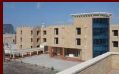
Operations office and Canteen Building
