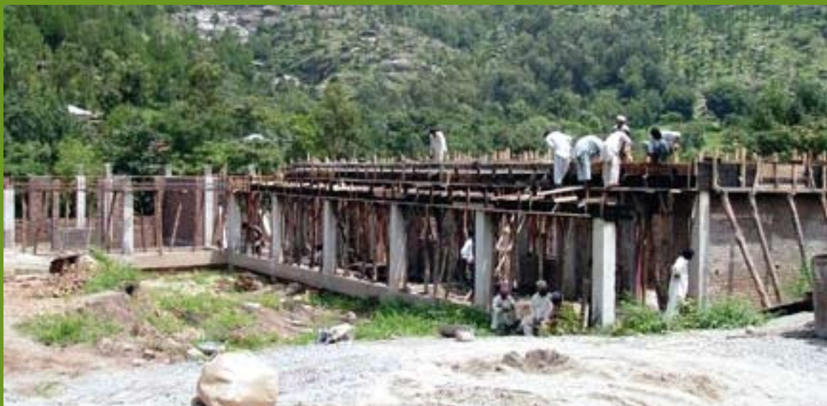
Reconstruction of a Primary School at Kandi in progress
